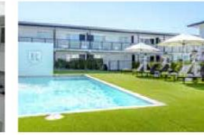
ROTORUA Regent of Rotorua Boutique Hotel
